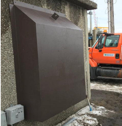
Installed shroud on the drawbridge's building housing the emergency generator
